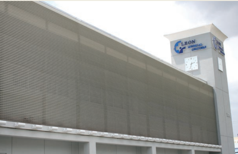
◀ Leon Medical Center, Miami FL, used aluminum louver as a sunshade to reduce solar glare and cooling costs.
