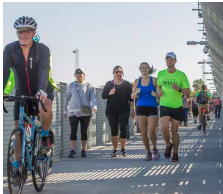
Big River Crossing in Memphis, TN (Aluminum Plank)
